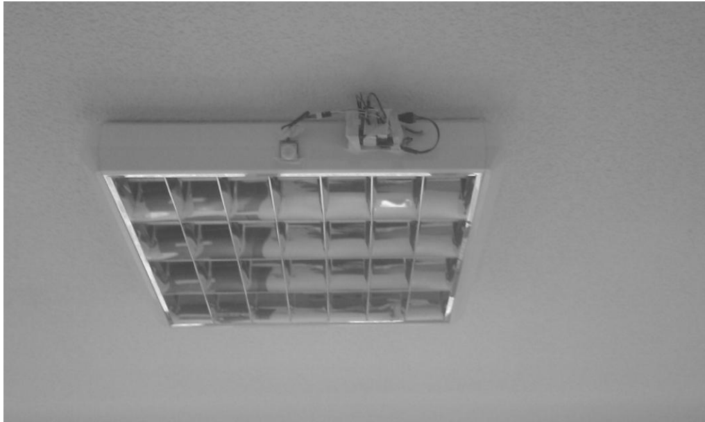
Figure 4.8- Prototype Implementation In Wireless Lab-Ceiling
