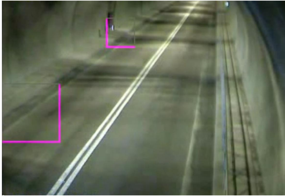
Figure1: Typical tunnel camera installation field of view (FOV)
