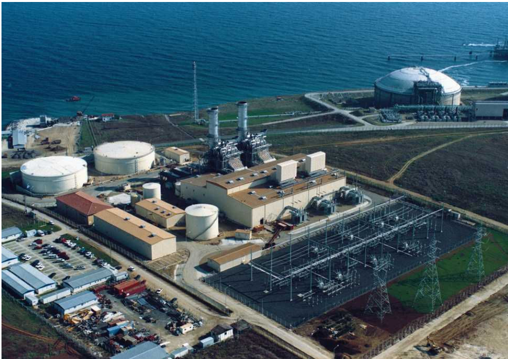
. Figure 1: A Combined Cycle Power Plant
