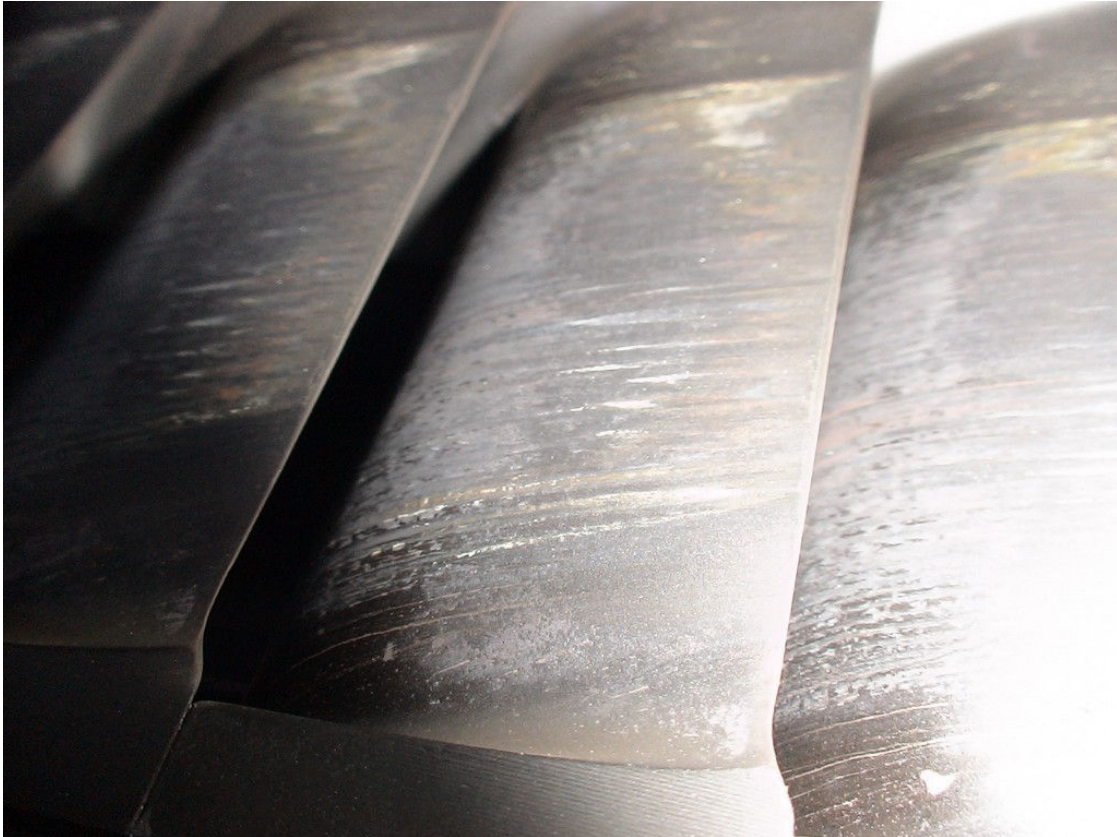
Figure 35: Eroded Steam Turbine Guide Vanes
