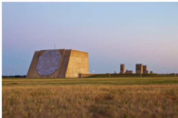
Figure 5: Passive Phased array example: AN/FPQ-16 [3]
