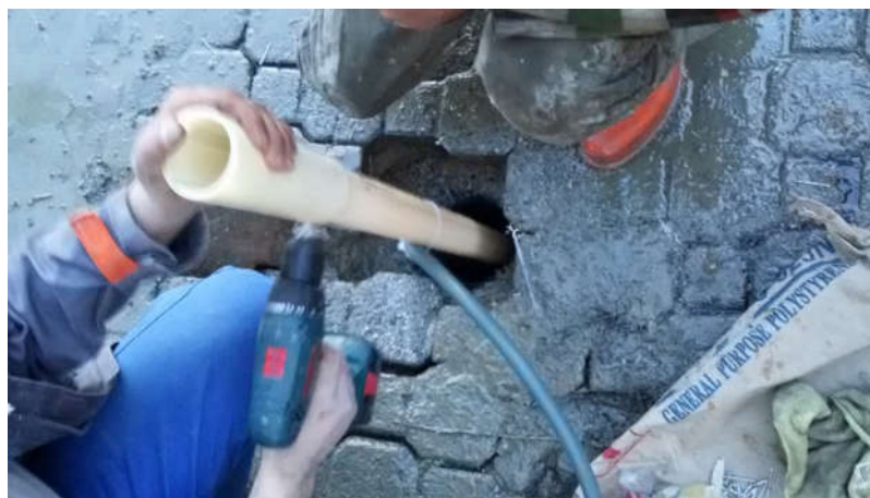
Figure 3.12: Field studies when placing the inclinometer tubes.
