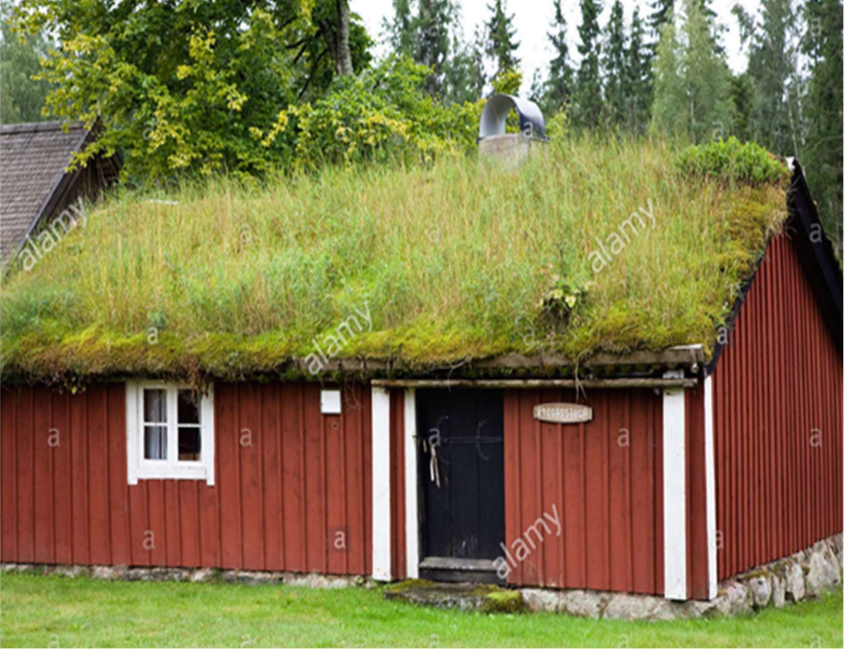
Şekil 4.7: Güney İsveç – Smaland’da yeşil çatı uygulaması ( https://www.alamy.com/stock-photo-typical-swedish-house-with-green-roof-smaland-south-sweden-scandinavia-48761158.html )
