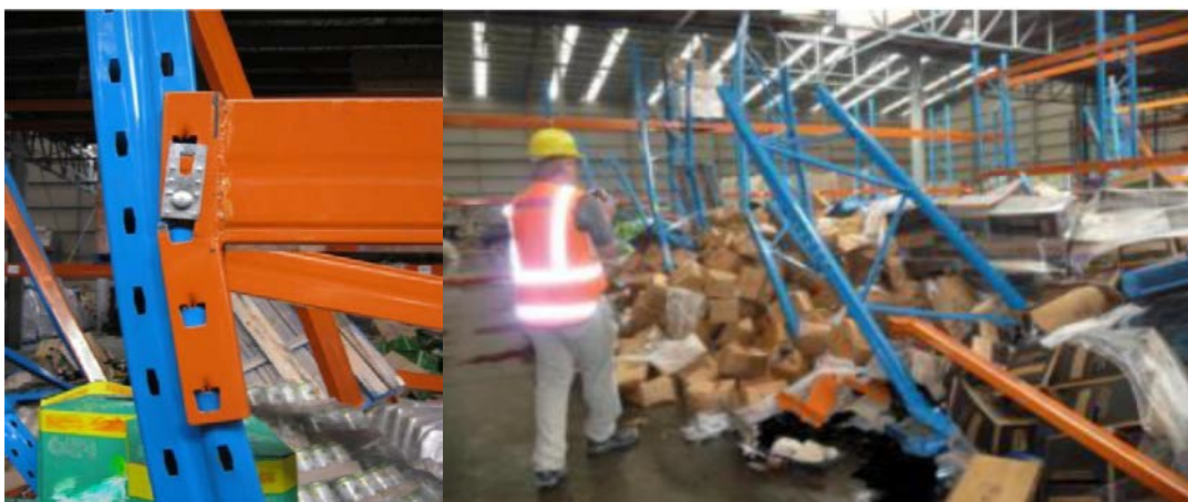
Figure 1.5: Collapsed rack system in Christchurch earthquake in 2011 (Clifton et al., 2011).
