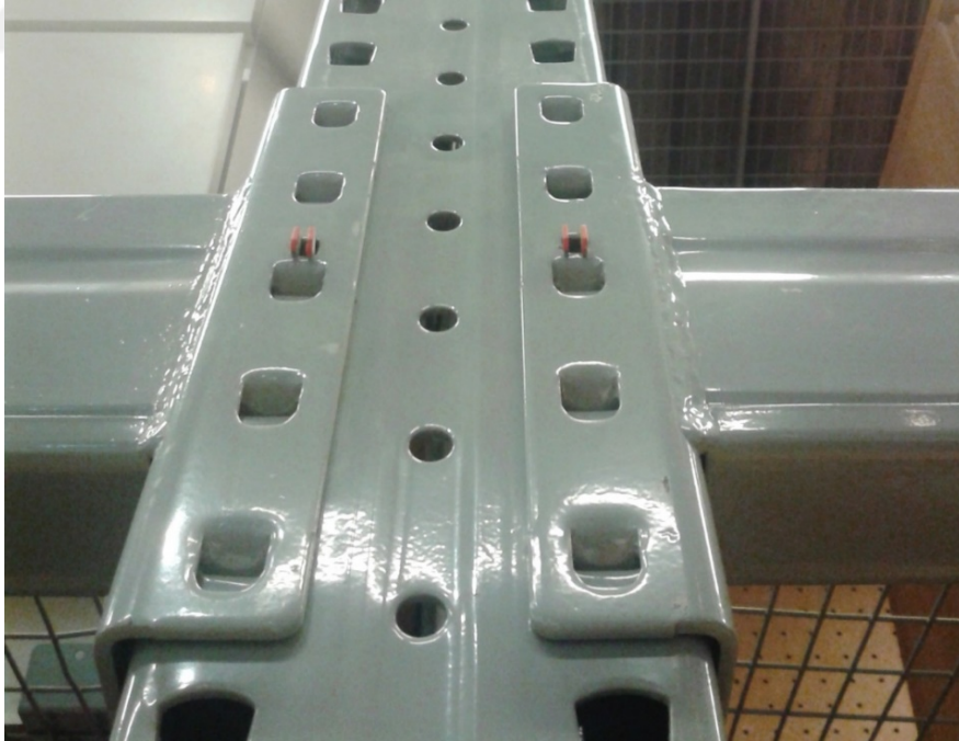
Figure 1.4: Beam-column connection (Elkadi, 2015).
