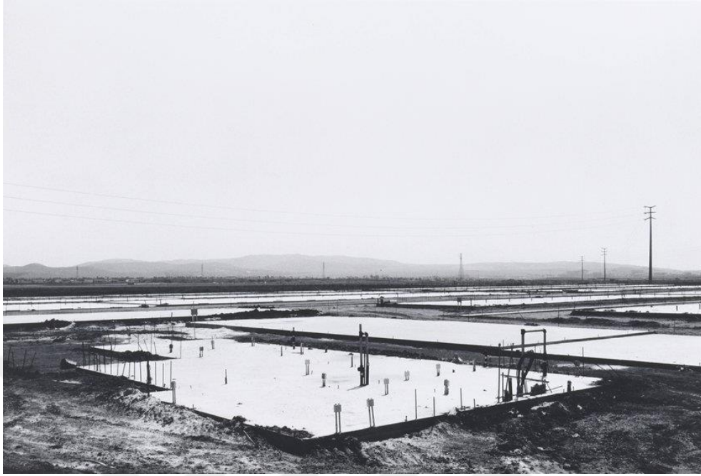
Görsel 3.24 Foundation Construction (1974) Lewis Baltz
