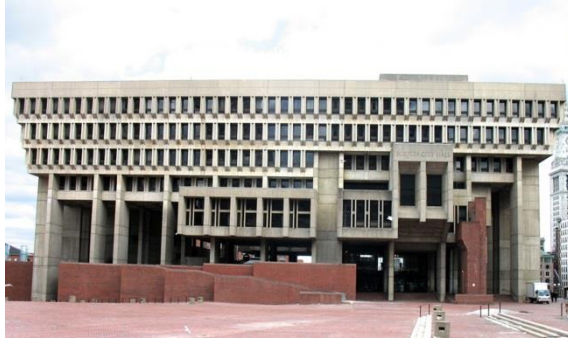
Resim 9 Boston City Hall, 1968, Michael McKinnell, Gerhard Kallmann, Boston
