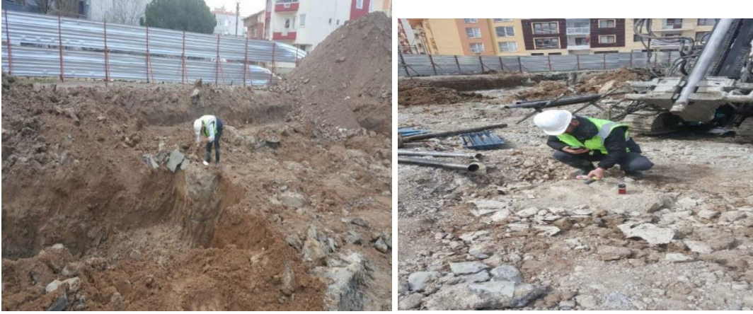
Şekil 3.19. Jet Grout Bütünlük Deneyi ( http://www.zeminarastirma.com/referanslar/canakkale-jet-grout-pit-sureklilik-deneyi/canakkale-jet-grout-butunluk-deneyi-pit-1/3/ )
