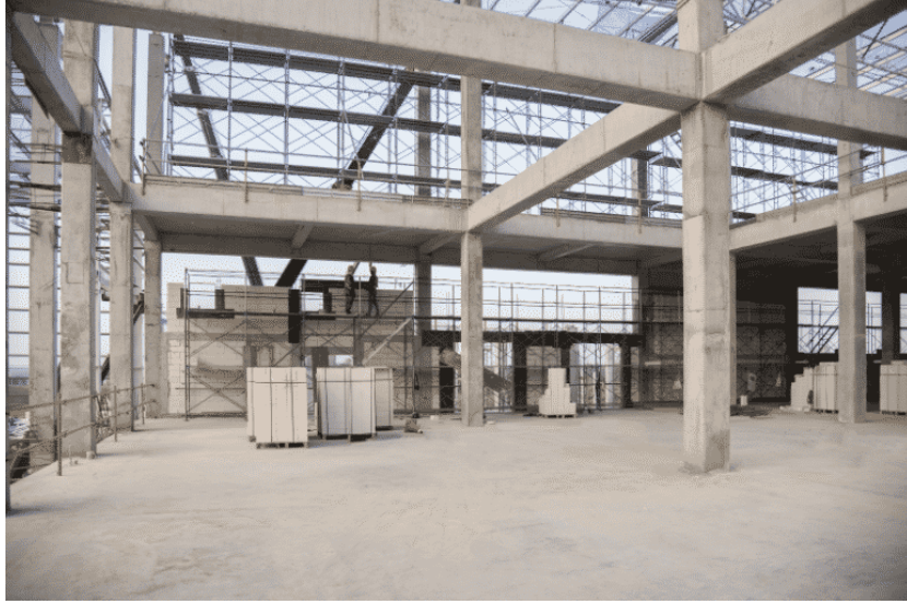
Şekil 3.2. Betonarme çerçeve sistem ( https://structuralengineeringbasics.com/what-are-beams-and-columns-building-construction/ )
