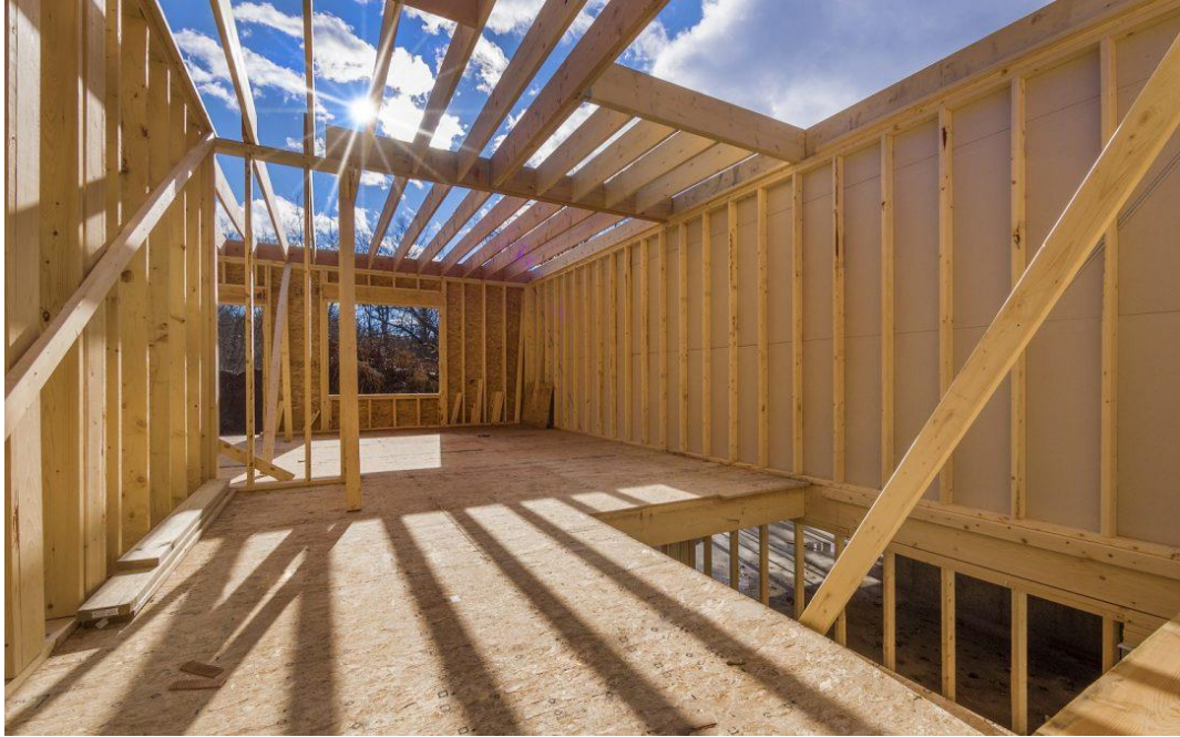
Şekil 3.1. Ahşap çerçeve sistem ( https://seagatestructures.com/common-misconceptions-of-wooden-building-construction/ )
