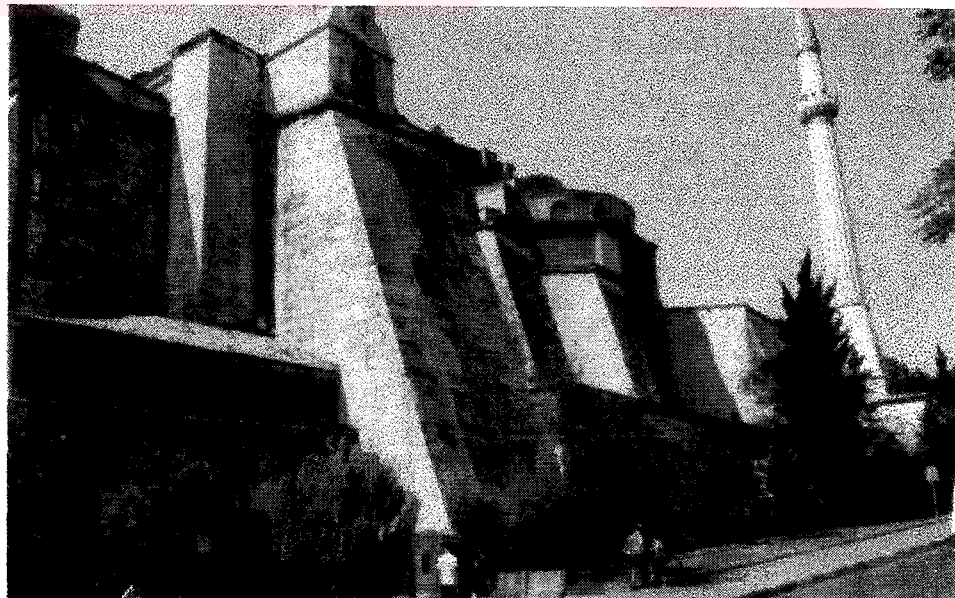
Figure 3.4-5 The Flying Buttresses at the East
