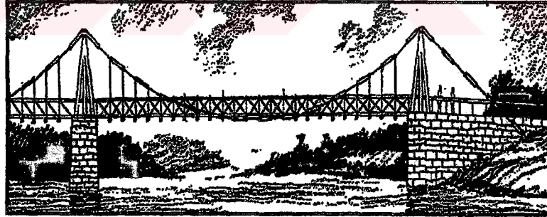
Şekil 3.79: Uniontown Köprüsü, James Findley, Uniontown, 1801
