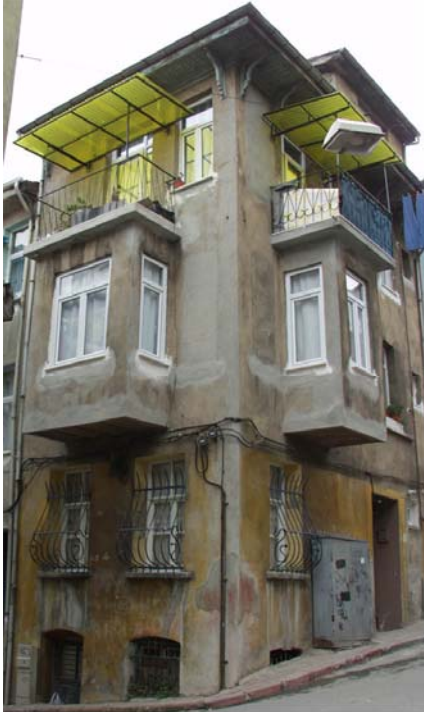
BEFORE RESTORATION / RESTORASYONDAN ONCE
