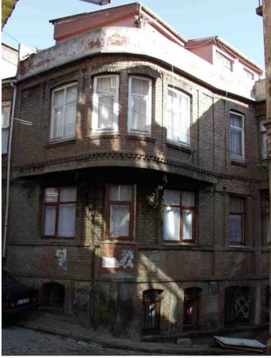
BEFORE RESTORATION / RESTORASYONDAN ONCE
