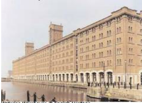
Waterloo Warehouse © English Heritage
