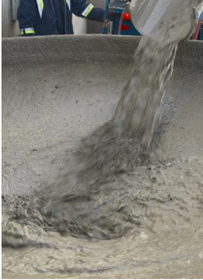
ekil 3.6 Haz,r beton kar, ,m,.
