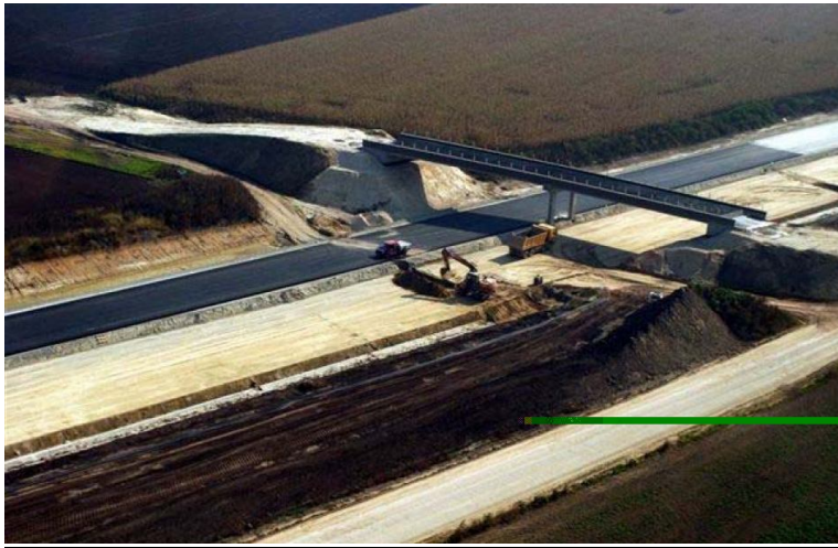
Picture 2.1 M6 Motorway (Schlor, 2006)
