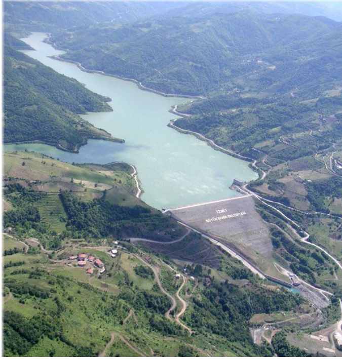
Picture 3.1 General view of İzmit-Su Dam ("Yuvacık Barajı'na", 2009)
