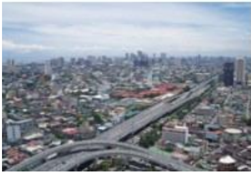
Picture 2.4 North Luzon Expressway ("North Luzon ", 2009)
