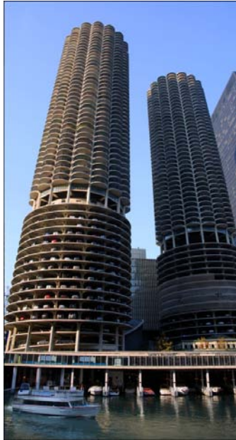
Şekil 2.29. Marina City Towers, 1964-67, Chicago
