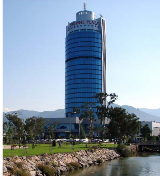
Şekil 2.54. Özdilek Crowne Tower, 2002, İzmir
