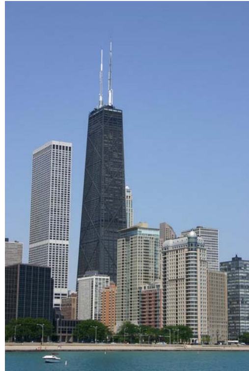
Şekil 2.27. John Hancock Tower, 1969, Chicago
