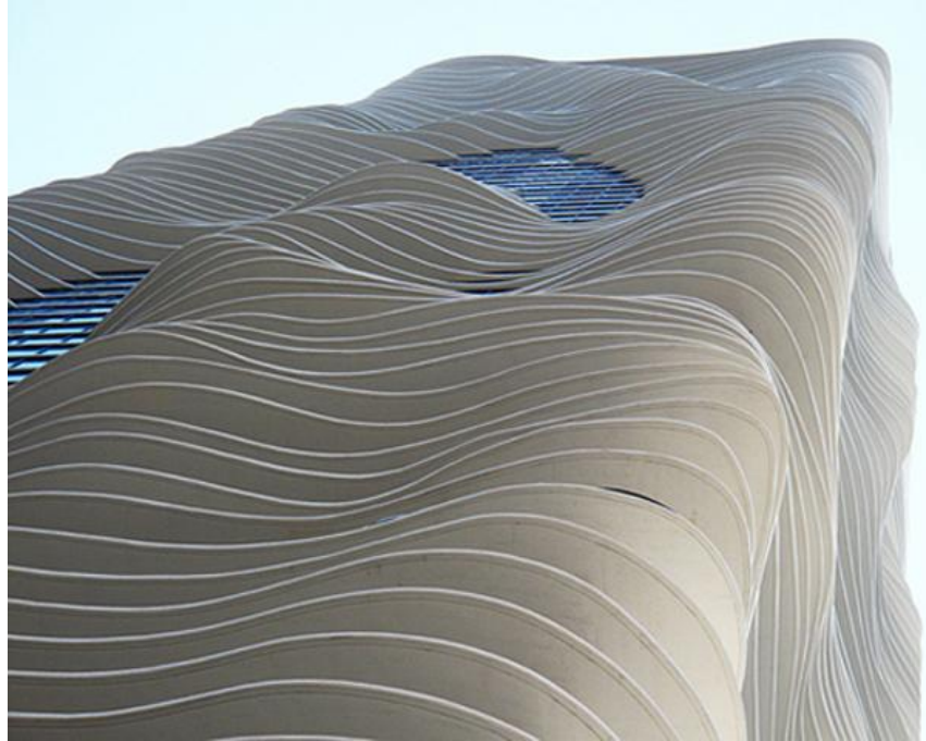
Şekil 4.164. Aqua Tower, Chicago, USA, 2008 409
