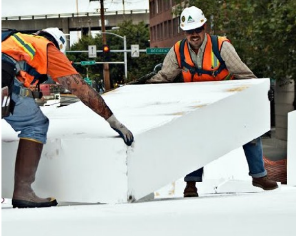
Şekil 2.56. Geofoam (wsdotblog.blogspot.com)
