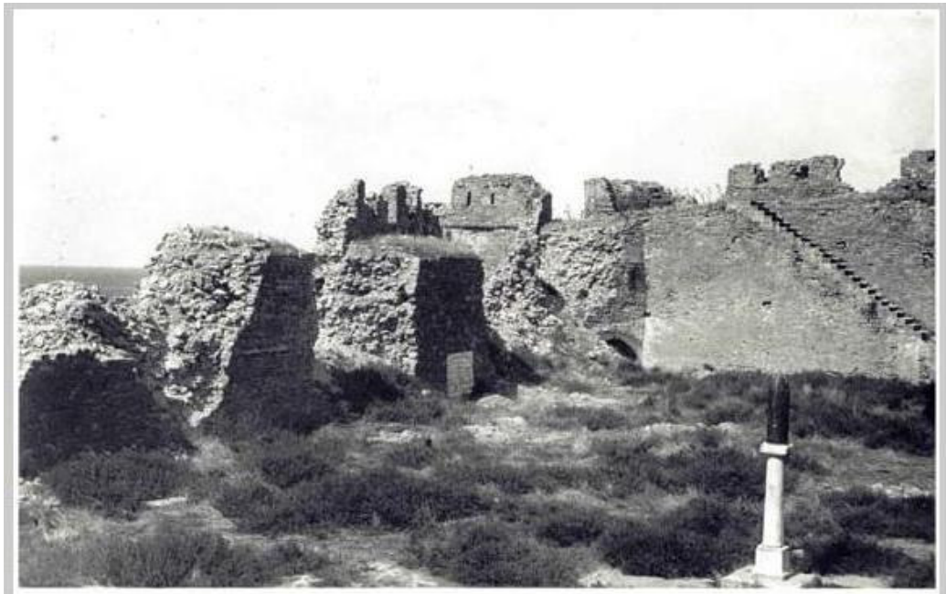
Image 9.19: The Southwest Wall during the wall from the upper courtyard, looking towards the southwest ( London Public Records )
