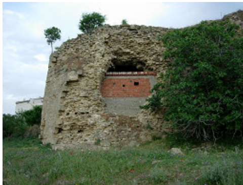
Image 9.13: The exterior façade of the North Tower ( Photograph courtesy of Kaletakımı )
