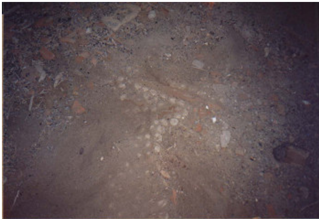
Image 9.47: Floor of the N. Tower, which was paved with inverted pinecones and brick in a radial shape (Photograph courtesy of Kaletakımı)
