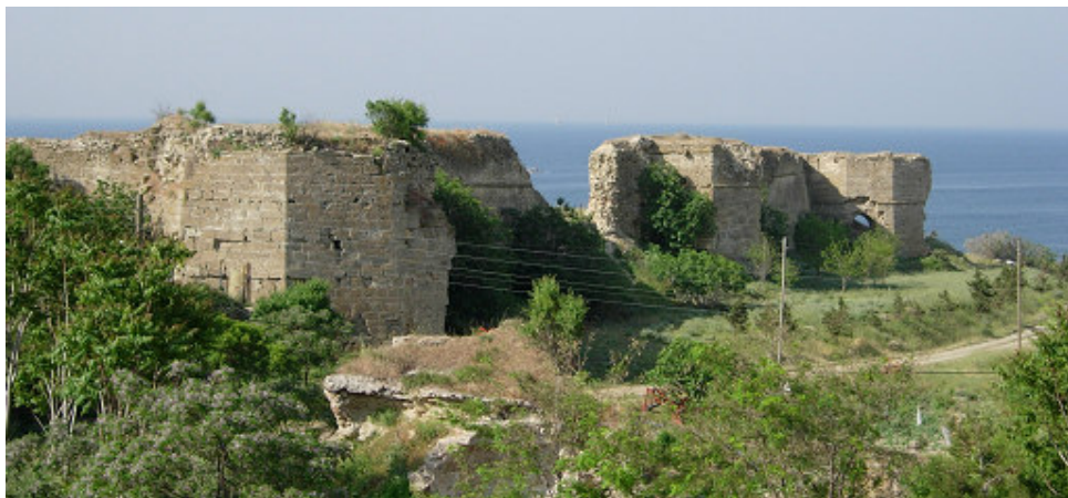
Image 9.11: The North Tower, Northwest Middle Tower and West Tower. Exterior (Photograph courtesy of Kaletakımı).
