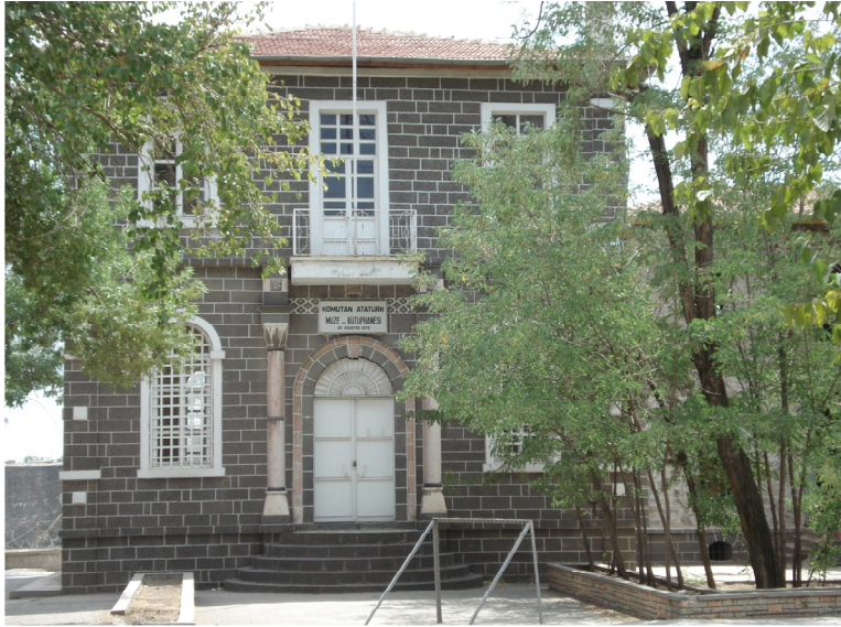
Figure 8: The already restored Atatürk Museum and Library, Information Center.
