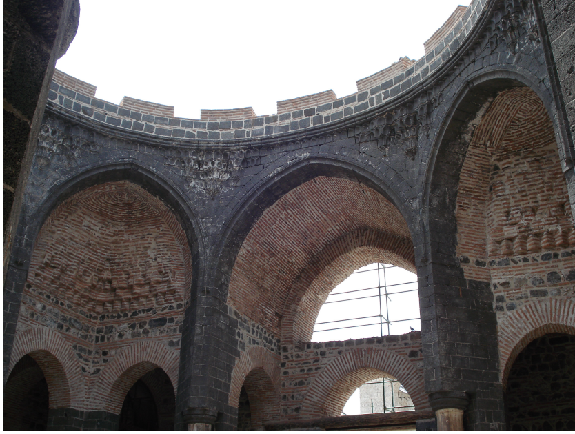
Figure 6: The entrance of the church of Saint George, a large square space to be covered by a dome.
