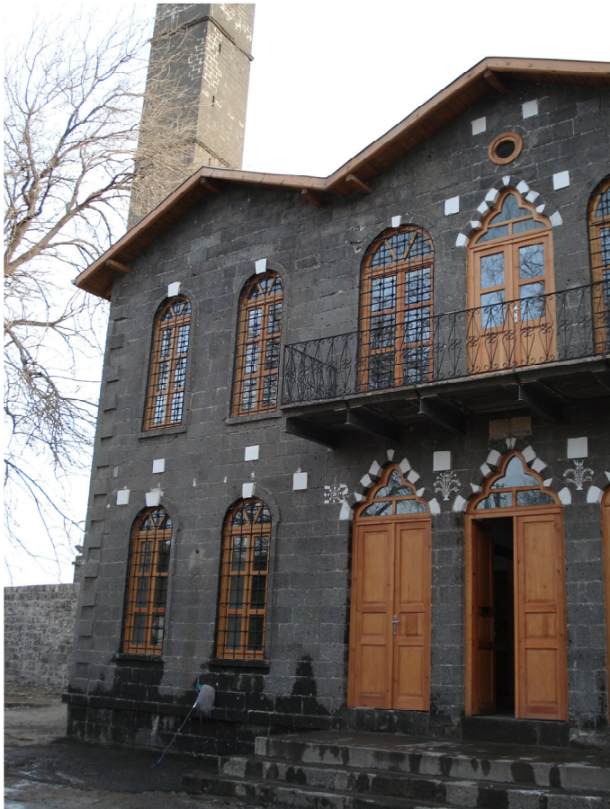
Figure 9: The Directorate of the Ministry of Culture and Tourism, with the typical Diyarbakır architecture alternating black basalt stone with white plaster decoration.
