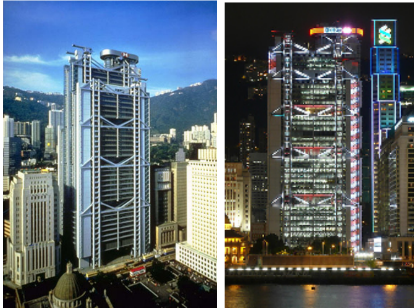
Figure A.4. Hongkong and Shanghai Bank (HSBC) Headquarters, Hong Kong 302
