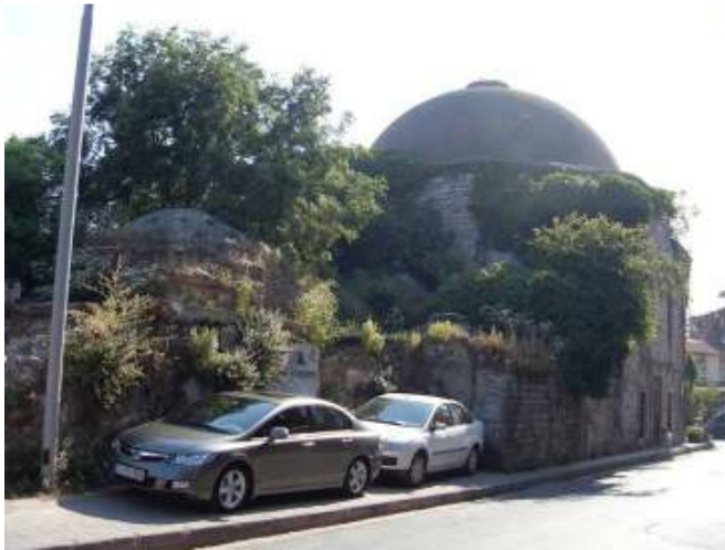
Fig. 18. (left) The Çardaklı Hamam
