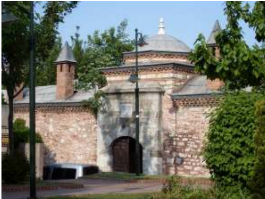
Fig. 24. The western entrance to the Küçük Ayasofya zâviye/medrese, look from the west
