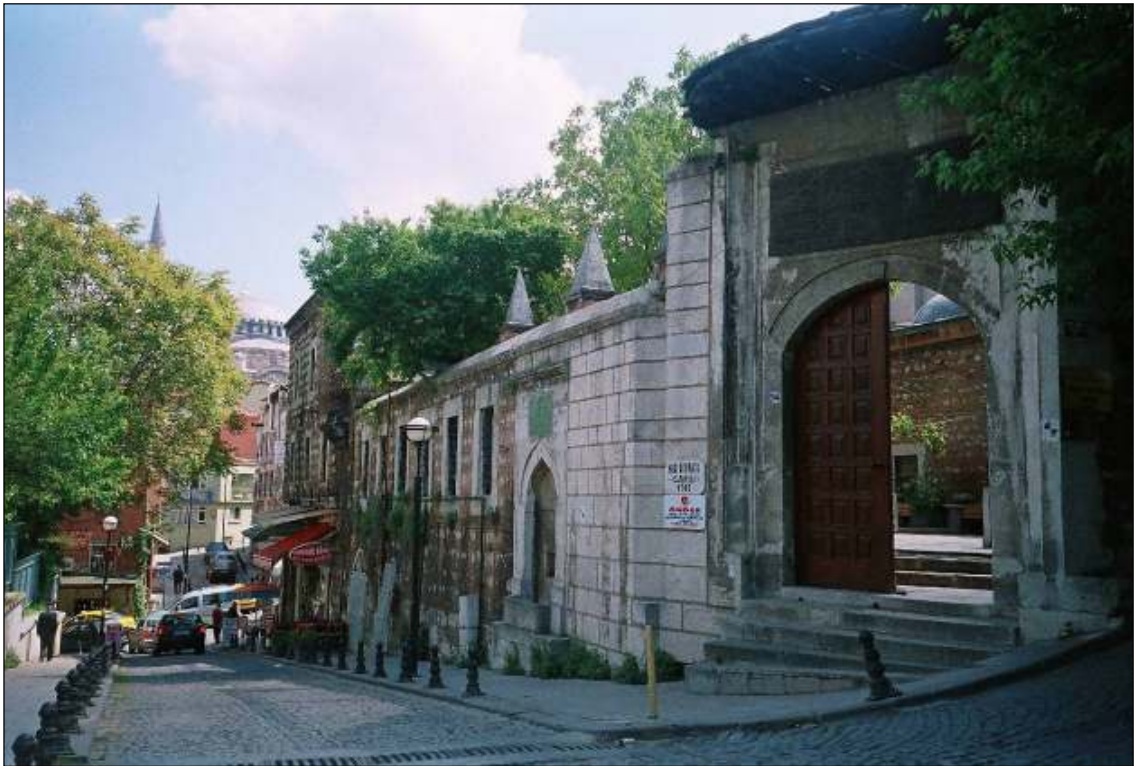
Fig. 48. Entrance of the Beshir Agha mosque complex and the view from the slope of Hükümet Konağı Caddesi towards Hagia Sophia
