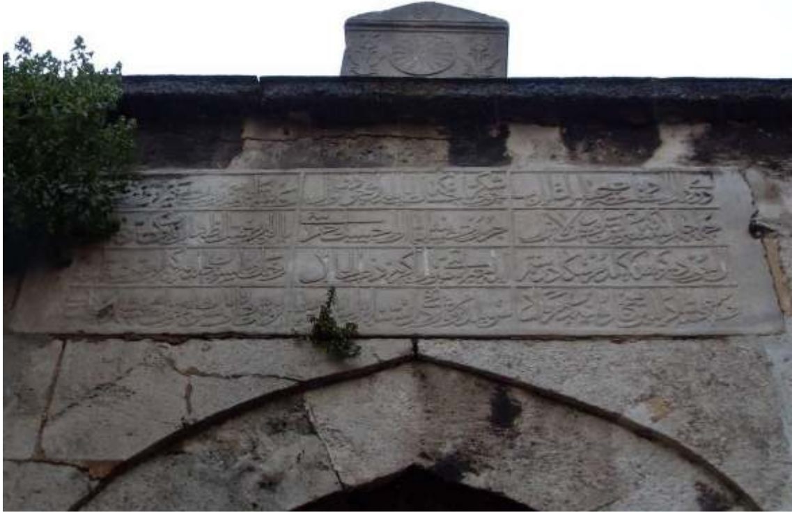
Fig. 47. The inscription of the fountain next to the Abbas Agha Mosque
