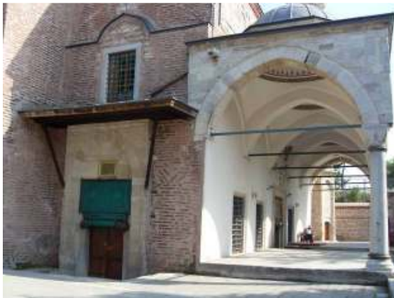
Fig. 21. The remodeled northern gate and the portico of the Küçük Ayasofya Mosque
