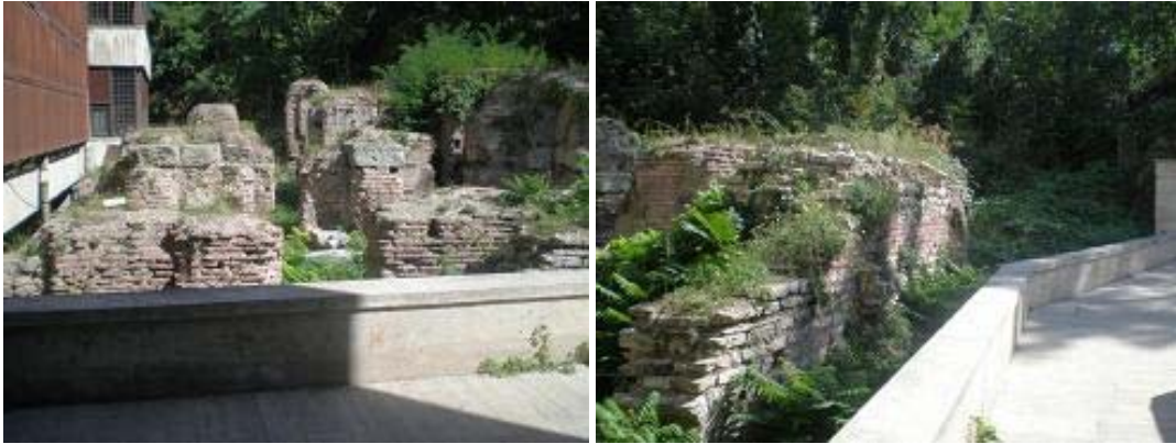
Figures 8.1 - 8.2 Views of the cistern from the balcony (Photographs by M. Bige Varlier)
