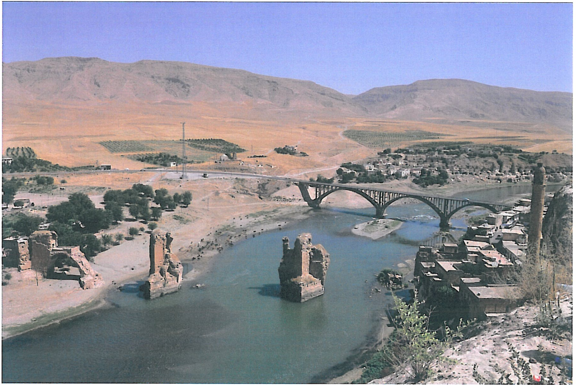
Photograph 1 Remains of the old bridge and the modern bridge.
