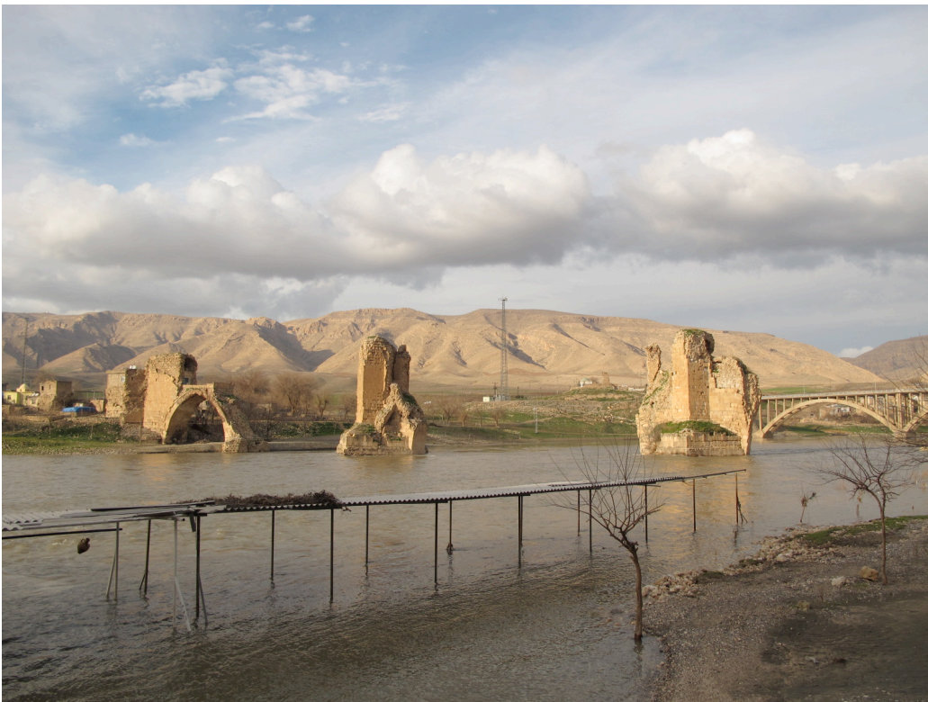
Figure 33. The Artukid Bridge
