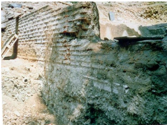
Fig 12 a: 6 th Century wall discovered during the excavations
