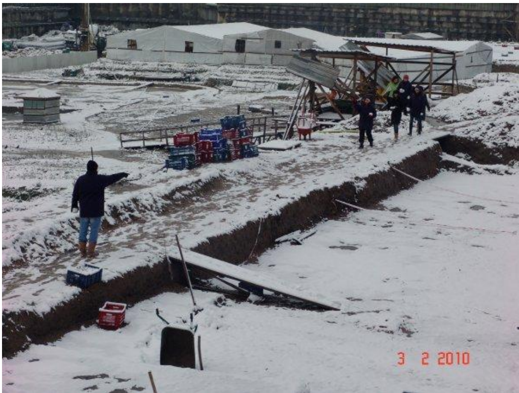
Fig. 27: View from the Yenikapı Excavation During the Winter
