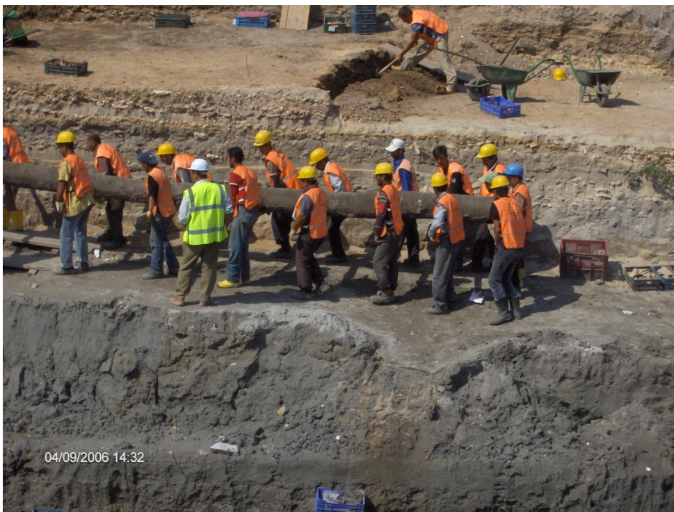
Fig. 23 b: Safety Equipments in Use
