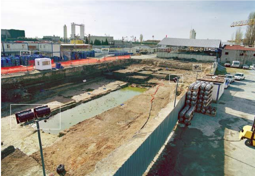
Fig. 30: Artificial Lightening Around the Trenches That Enabled the Night Shifts
