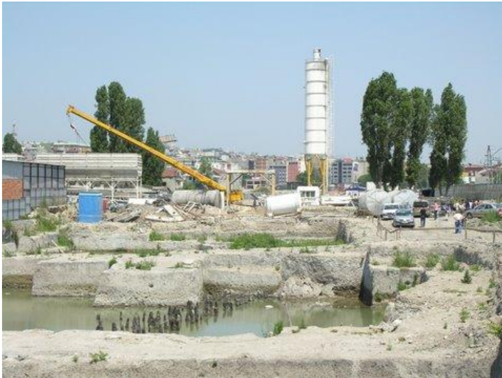
Fig. 25: Construction of the Concrete Plant at the Marmaray Excavation Site
