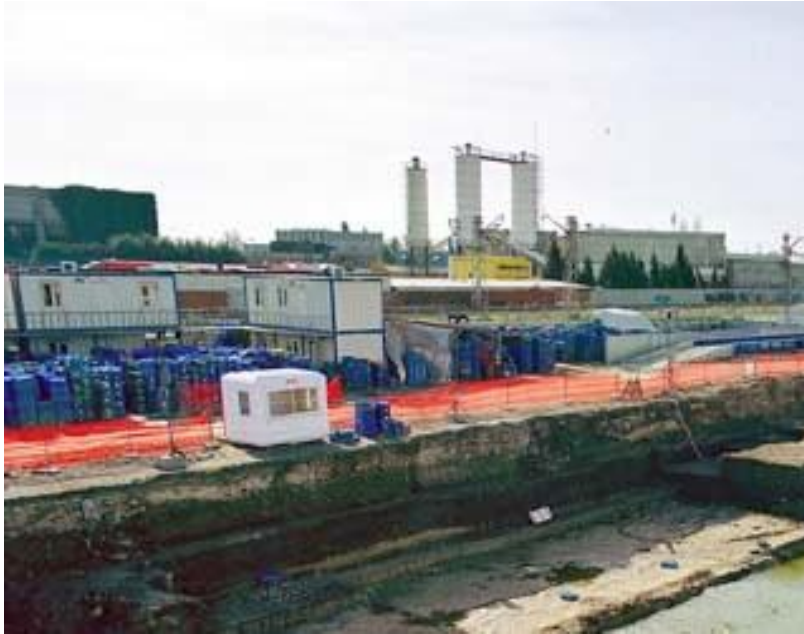
Fig. 28: Prefabricated Cabins That Were Used During the Winter
