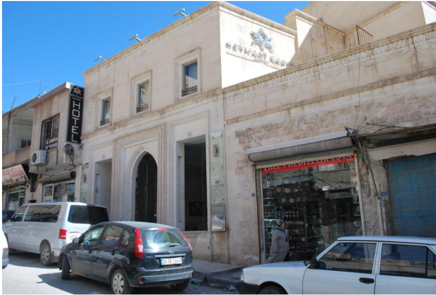
Figure 68 Newly constructed hotel, Mardin. March 18, 2012. Photograph taken by author. JPEG file.
