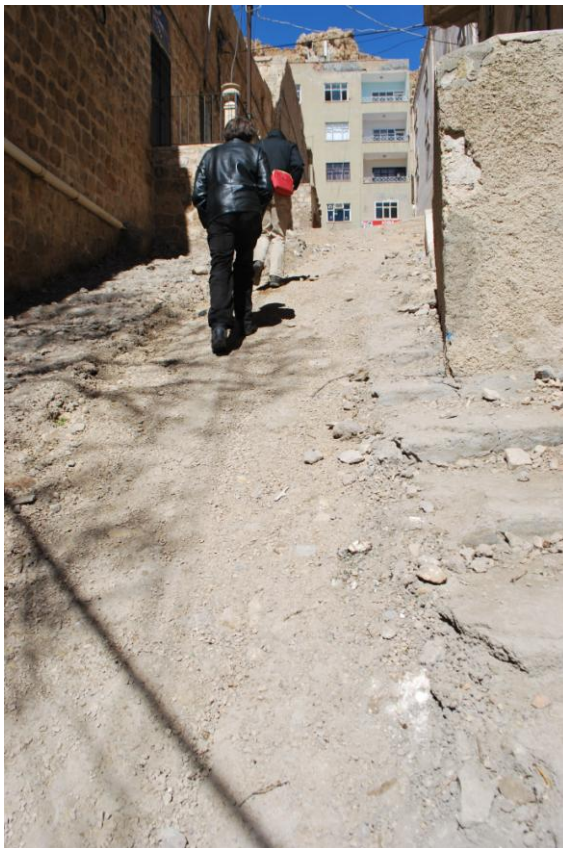
Figure 71 Street under construction, Mardin. March 18. 2012. Photograph taken by author. JPEG file.
