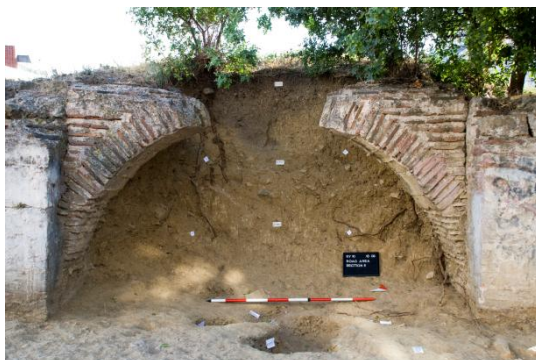
Figure 7. Detail from the northern wall showing the relationship between the arch and the buttress to the left, from the Küçükyalı ArkeoPark Project archives (2010).
