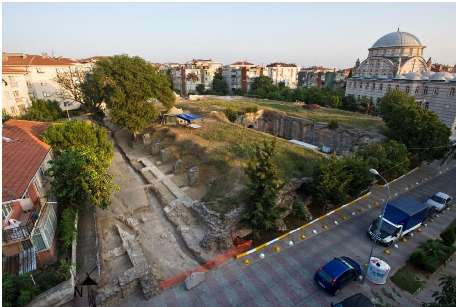
Figure 4. View of the western walls at Küçükyalı from the north. From the KAP archives (2010)
