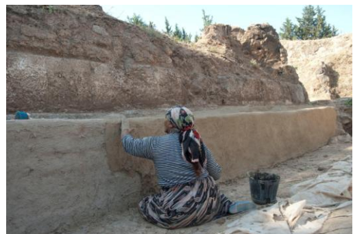
Photo 20 Plastering Phase of the Mud Brick Wall (Courtesy Murat Akar)
