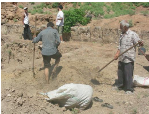
Photo 17 Preparing the mud and straw mixture
