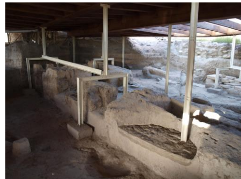
Photo 11 Adobe blocks and metal harnesses supporting the structure at Arslantepe (Courtesy of Ben Classz Coockson)
