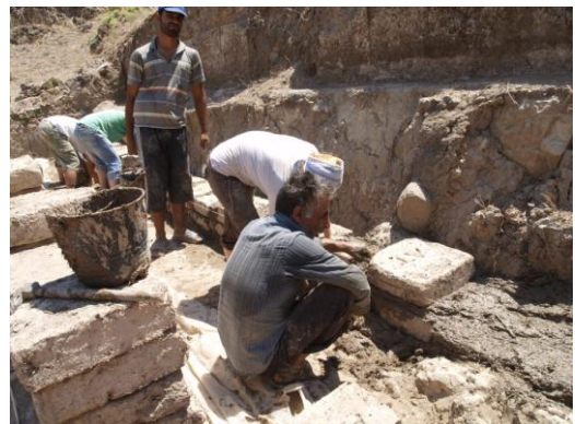
Photo 18 Laying the new mud brick wall
