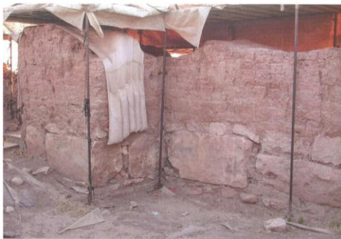
Figure 8 Detail of the protective structure over the remains at Tell Mozan/Urkesk (Buccellati 2006a in Agnew and Bridgeland 2006: 76)
