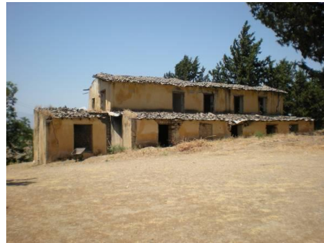
Photo 65 Woolley’s Dig House, Back, current state as of 2010
