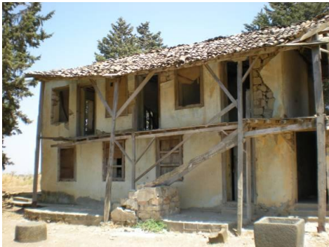
Photo 64 Woolley’s Dig House, front, current state as of 2010
