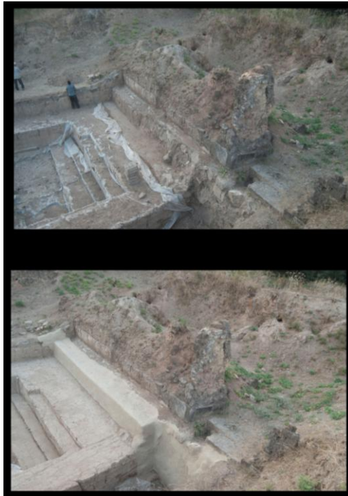
Photo 16 Before and After of the Restoration Project (Murat Akar)
