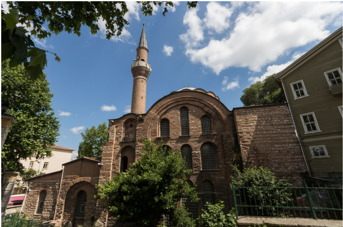
Figure 2: Exterior view from the northwest (June 2016 - Photo Kaan Dönbekci)
