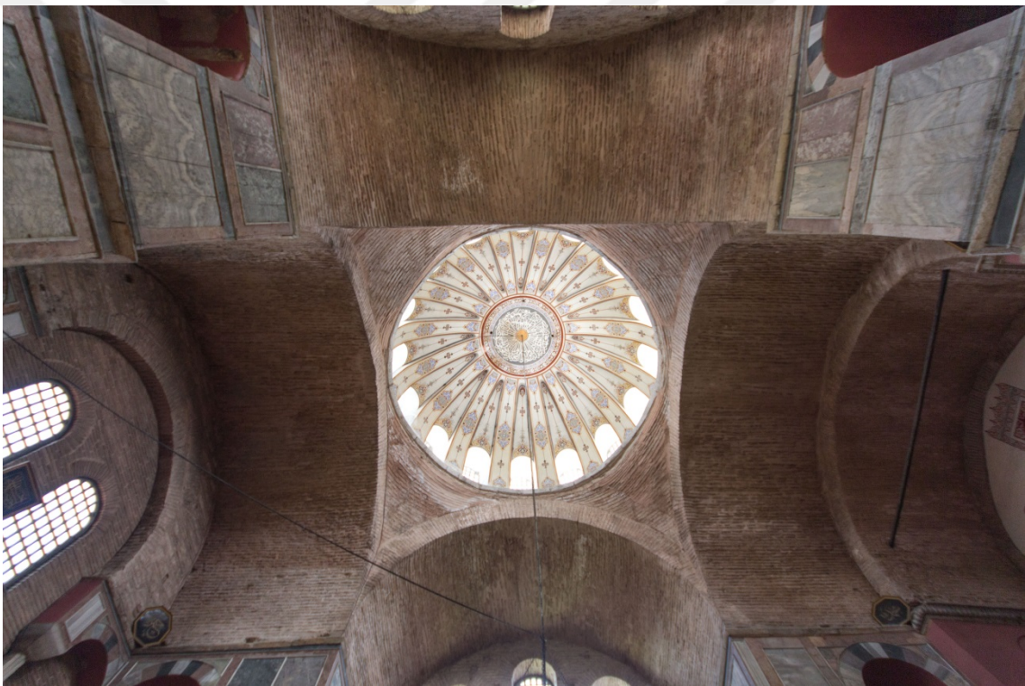
Figure 13: Interior view of central dome (June 2016 - Photo Kaan Dönbekci)
