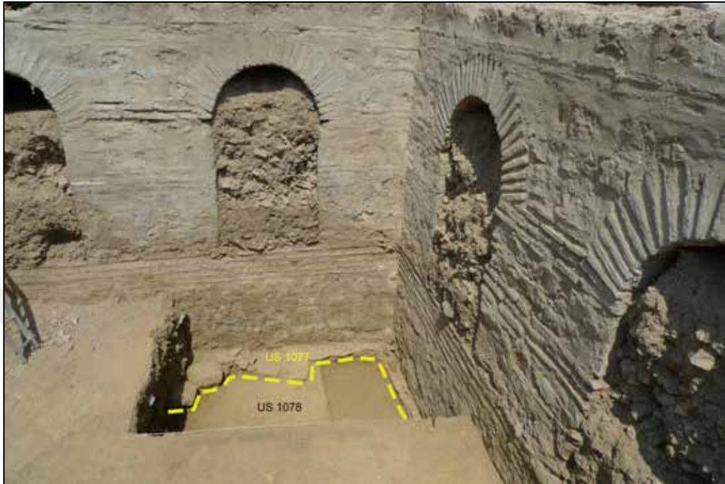
Fig. 6: Tower. Trench by the N-corner, showing foundation (US 1077) and the adjoining layer (US 1078) [KYAP 2010, with additions by the author].
