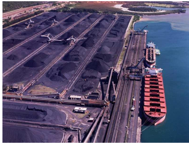
Figure 4. A typical bulk port stockyard
