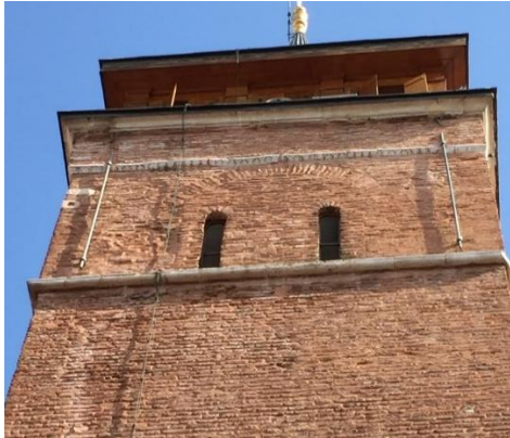
The Middle Byzantine cornice in the upper part of the belfry, the Arap Camii. Photograph by the author, 16.10.2018.
