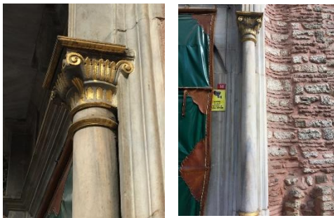
The gilded Ionic capital on the marble column in the southern portal, the Arap Camii.
