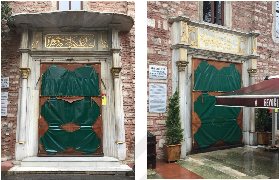
The portals of the Arap Camii.
