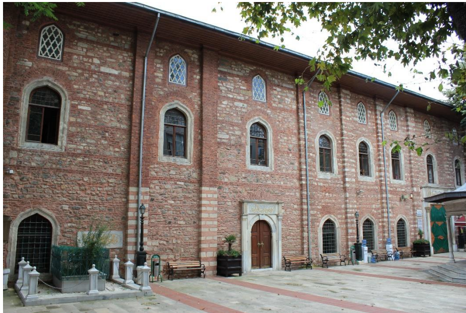
The brick and stone masonry of the Arap Camii.
