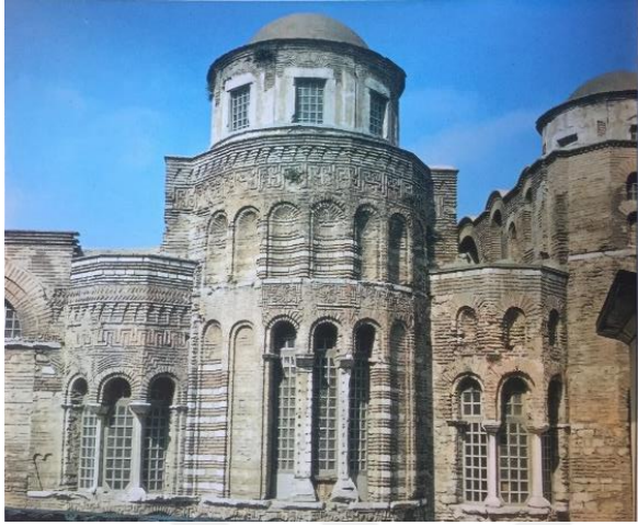
Monastery of Constantine Lips, (Feneri İsa Camii), view of the exterior, Istanbul. Mango, Byzantine Architecture , 150.
