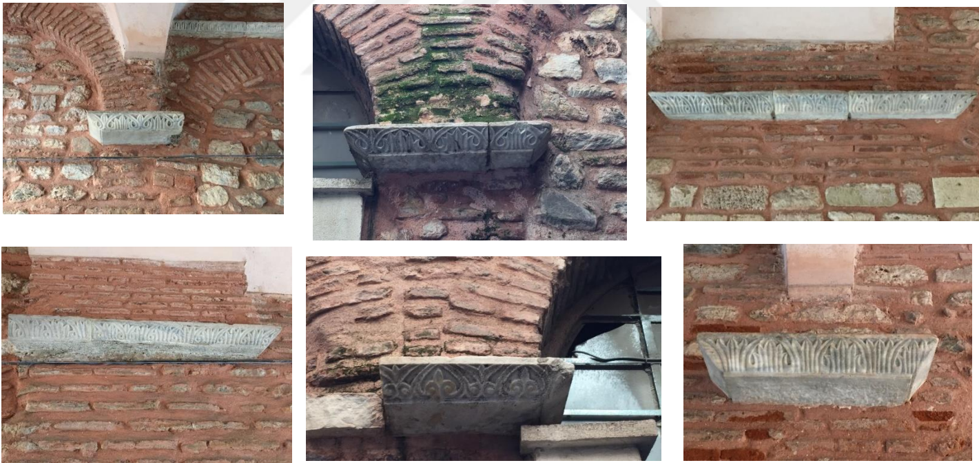
The impost capitals in the tower passage, with lotus and palmette friezes in Middle Byzantine style, the Arap Camii.
