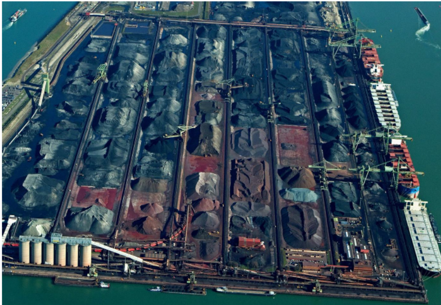
Figure 1.5: A stockyard with lanes and separated piles
