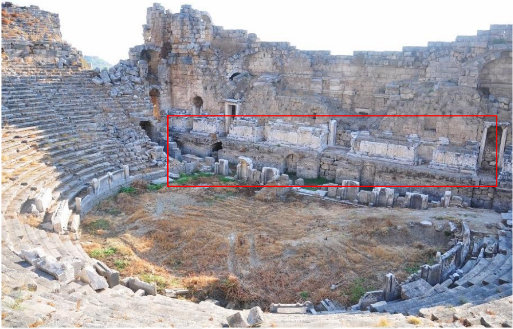
4.209: Theater of Perge and the Dionysiac frieze on the stage building (Perge Excavation Archive).
