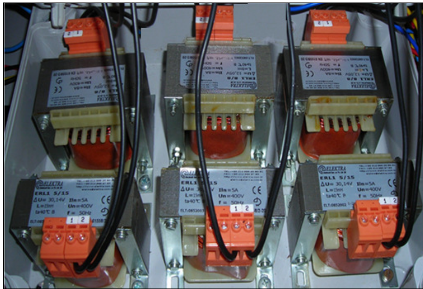
Figure 6.14. Choke reactors (on the top) and interface reactors (on the bottom)
