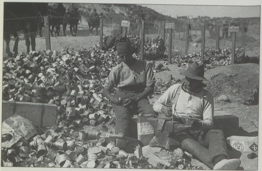
25. A chronic shortage of grenades forced the British and Anzac troops to improvise by using precariously fuzed jam tins filled with scrap metal and an explosive charge. 'Grenade factories' such as this one at Anzac were set up. In this case the manufacturers, with cheerful disregard for any evident safety precautions, are using a metal punch and anvil to prepare the tins for filling, whilst a mule train passes close by, oblivious to the risk of spontaneous detonation
