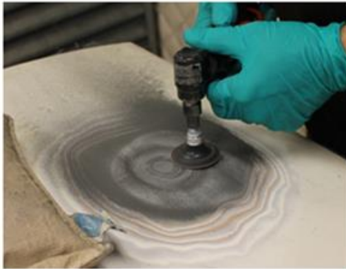
Figure 3.6: Scarf Repair taper laminate removal example 1.
