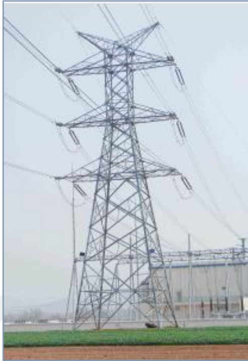
Figure 2.9: A steel lattice tower
