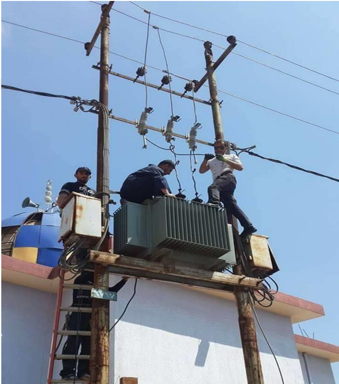
Figure 4.4: Changing the naked wires by other one insulated.
