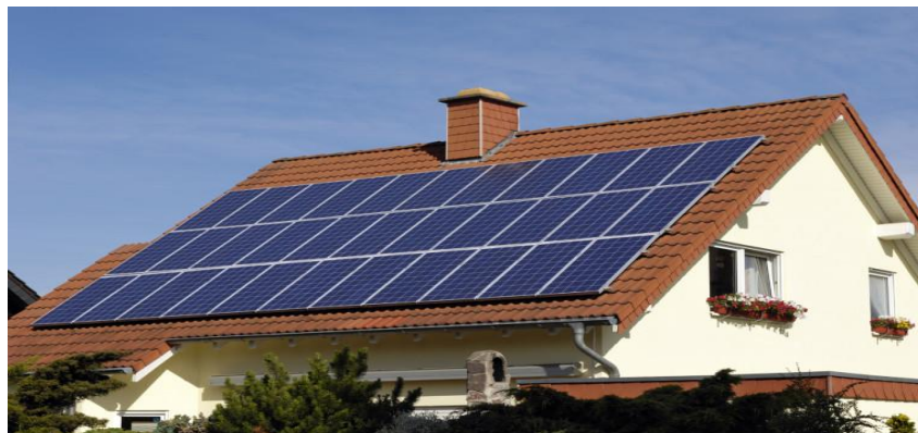
Figure 2.11: Photovoltaic panels in homes.
