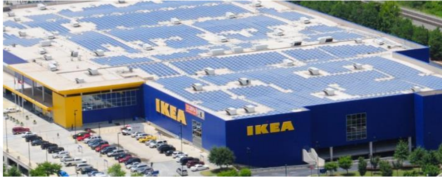
Figure 2.12: Photovoltaic panels for commercial usage.
