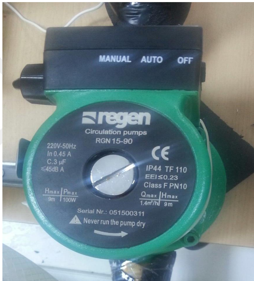
Figure 3.6: The hot water Pump.
