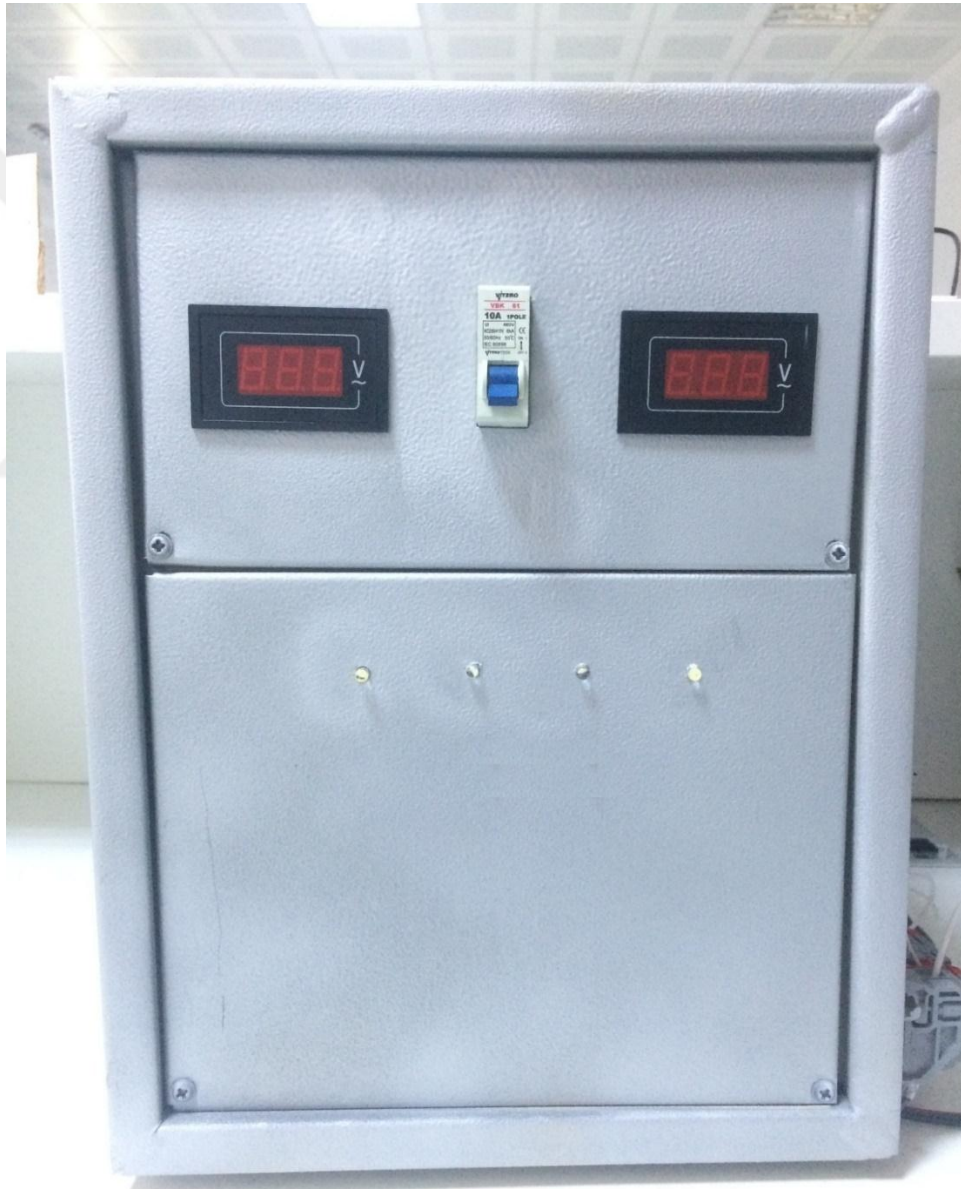
Appendix 1 : Front View
