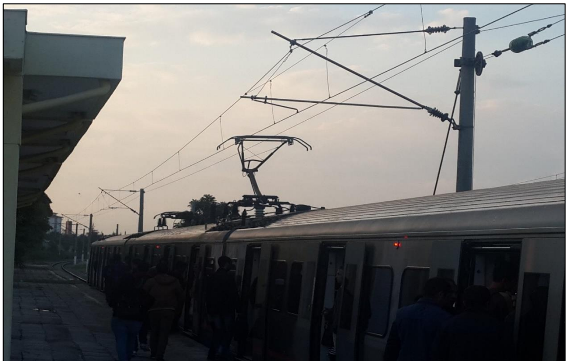
Figure 3.17: Overhead connection probe (This photo was taken by the researcher)
