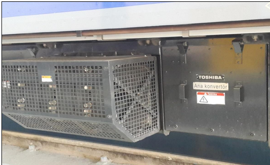
Figure 3.19: Main converter. (This photo was taken by the researcher)
