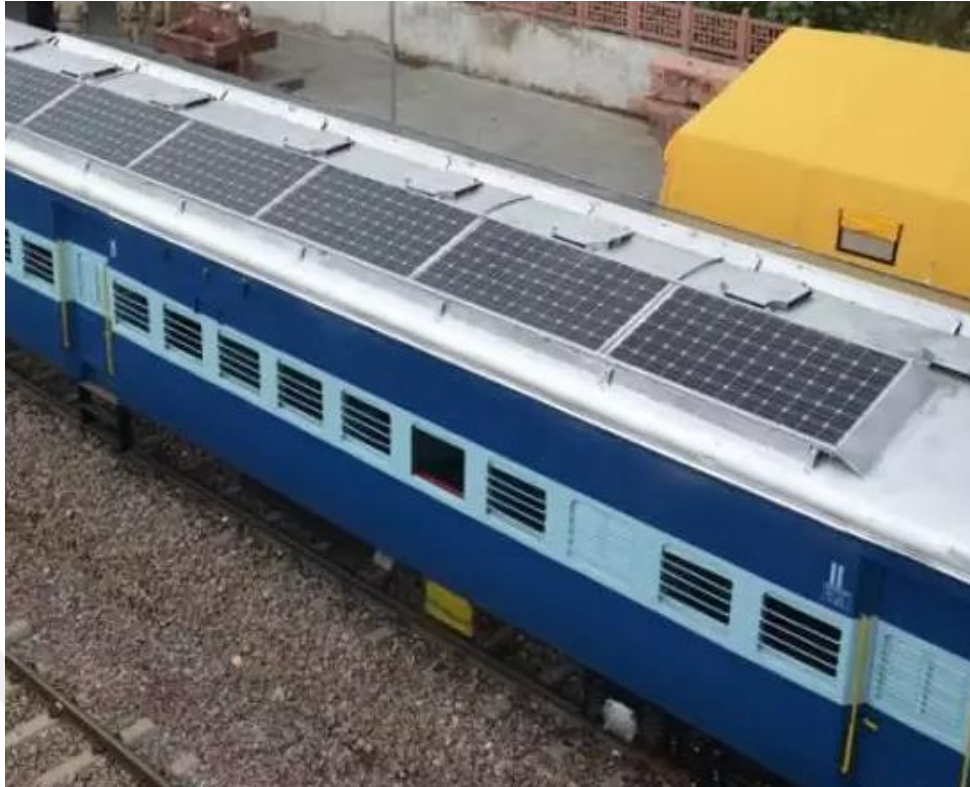
Figure 3.14: Train with solar panel on rooftop [32].
