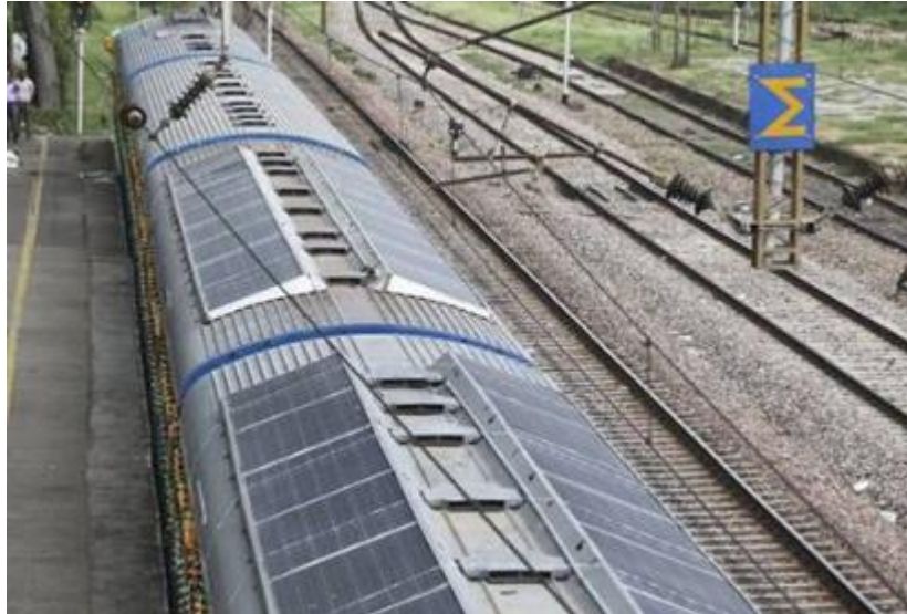
Figure 2.1: Solar photovoltaic system sample application of Indian railways [Singh, K. (2017)].
