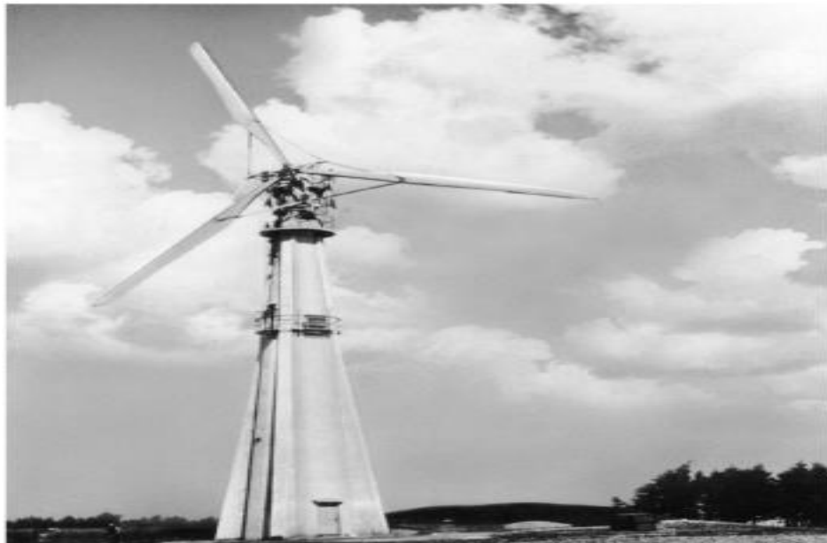
Figure.1.5. Smidth Turbine. (Three blades -Diameter 24m -Rated Capacity 70 kW), 1942 [6]
