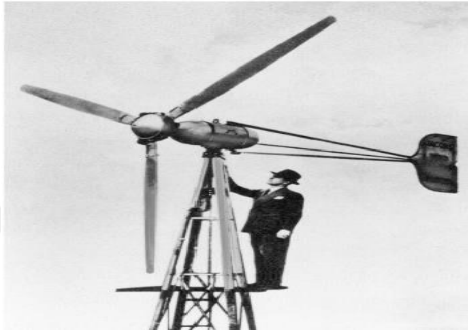
Figure 1.7. Jacob's "Wind Charger" (4m rotor Diameter, Rated Power 1.8 3kW), 1932
