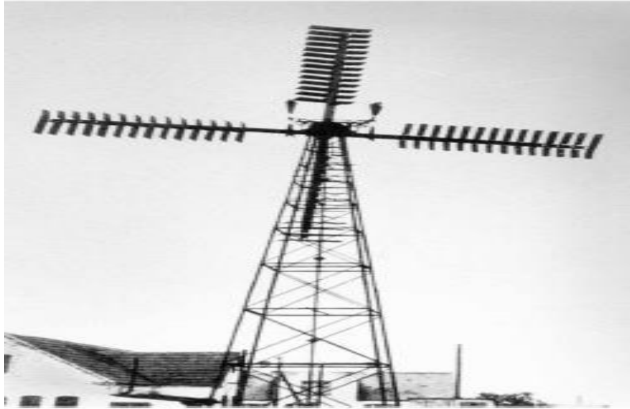
Figure.1.4. Turbine of La-Cour-Lykkegard (18m, 30kW and rated speed 12m/s) in Denmark [5]
