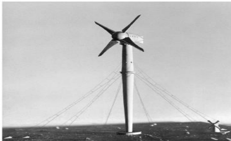
Figure.1.6. Project Kleinhenz Whit (130m Rotor Diameter and 10,000kW Rated Power), 1942
