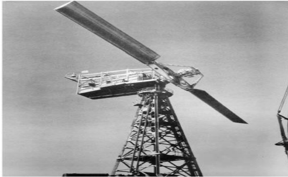
Fig. 1.8. Smith Wind Turbine, US: 53.2m Rotor Diameter 1251kW Rated Power (1941) [9]
