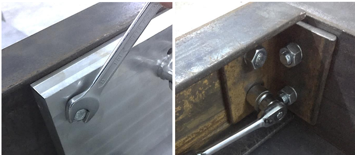
Figure 7.9: Daily control of bolted joint pre-tensions
