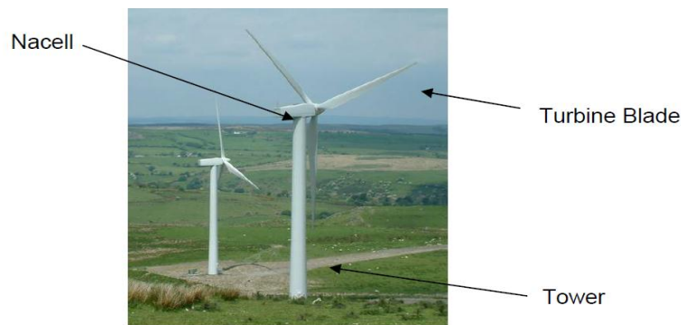
Figure 3.1 : Main parts of a standard wind turbine.
