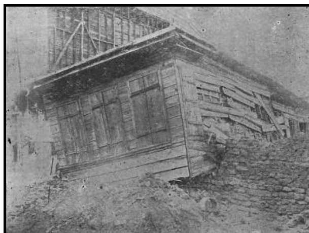
Figure A3.3 : A collapsed house at Tekirdağ, build of wood on top of bricks.
