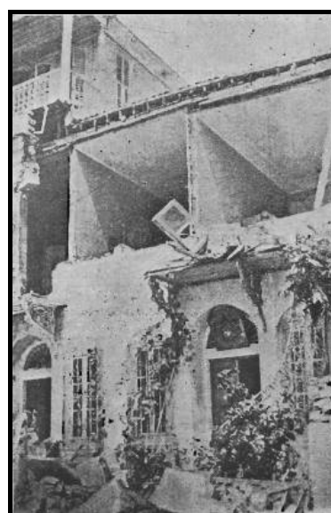
Figure A3.15 : Damaged building at Çanakkale (Sadi, 1912).
