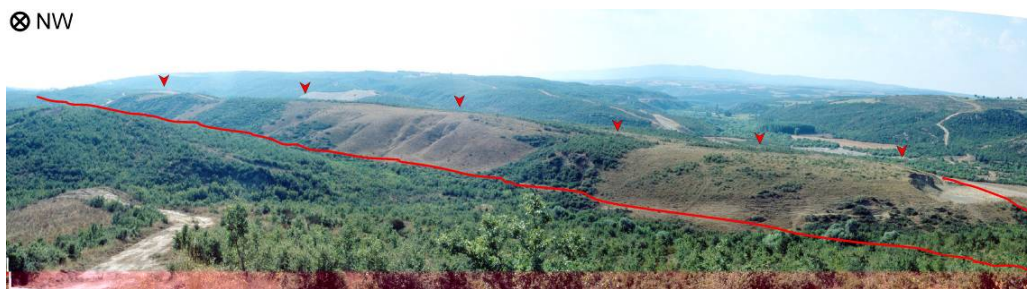
Figure 4.15 : A linear pressure-ridge west of Gölcük oriented 18^\circ oblique to the Ganos fault. It is bounded by strike-slip faults and rises as a push-up structure.
