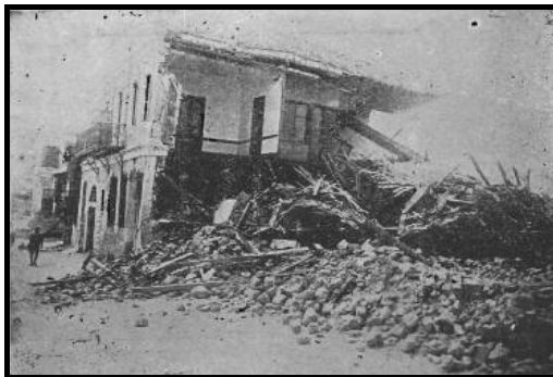
Figure A3.25 : Adjacent buldings of different type. The Stone building survived with slight damage, while the other was totally destroyed (Mürefte, Mihailovic, 1933).
