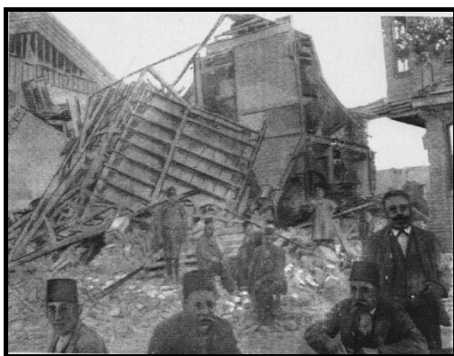
Figure A3.11 : Collapsed buildings at Şarköy (Sadi, 1912).
