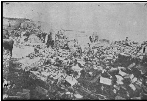
Figure A3.24 : The main road of Mürefte after the earthquake.
