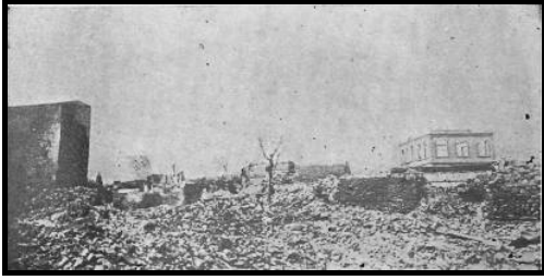
Figure A3.17 : Ruined main road at Ganos (Gaziköy; Mihailovic, 1933).
