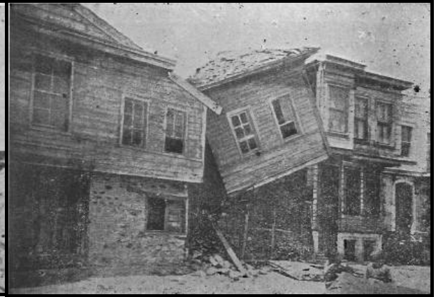
Figure A3.26 : A house, which wooden part tumbled to the side when the bricks underneath collapsed (Mürefte, Mihailovic, 1933).
