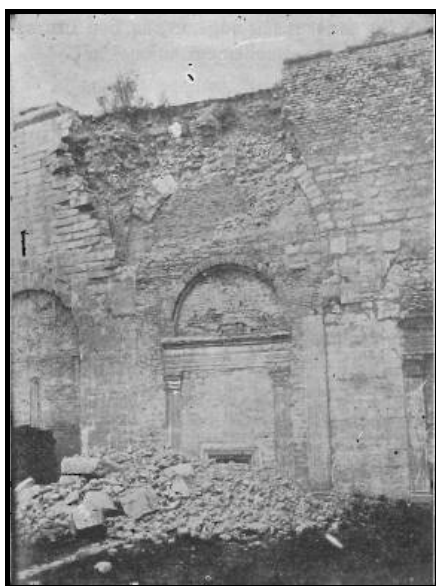
Figure A3.1 : Damage city walls at İstanbul (Mihailovic, 1933)
