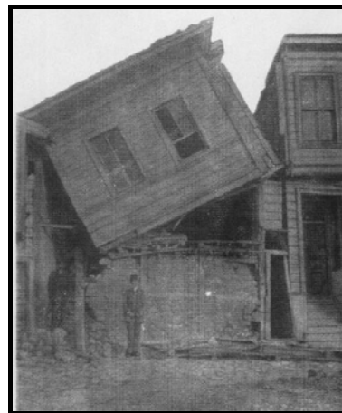
Figure A3.10 : Tumbled typical house of the region. Bottom of the construction is build by bricks, while the top is made of wood (Sadi, 1912).
