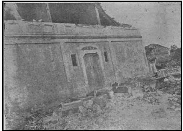
Figure A3.27 : Destroyed Stone building at Şarköy (Mihailovic, 1933).
